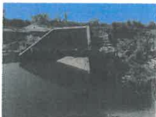
20) The 48" diameter RCP outlet, wingwalls, and footing at station LV 8+60 have fallen into a scour hole in the Salt Creek Floodway. See the structural drawings for final repair.
