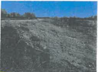
18) A 35 foot wide and 50 foot long area on the riverside levee slope was used as a ramp, killing the sod cover and damaging the top foot of topsoil. Mow and scarify the damaged slope and place 6 inches of levee aggregate surfacing.
