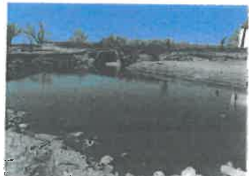
25) The drainage swale from the RC box culvert and 48" RCP drainage structures experienced areas of scour and deposition from the 2019 flood event that impacted its design elevation of 1056.0 feet NGVD29. Excavate floodway to elevation 1055.5, place 6 inches of topsoil to elevation 1056, and seed.
