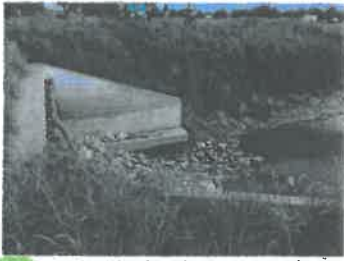
22) Approximately 8 feet of scour downstream of the reinforced concrete box culverts into the riverside levee section and BNSF berm for a length of 75 feet, leading to failure of the erosion control matting and large erosion gullies in the embankment slope. Additionally, there is 3 feet of scour underneath the wingwalls of the drainage structure. See the structural drawings for final repair.
