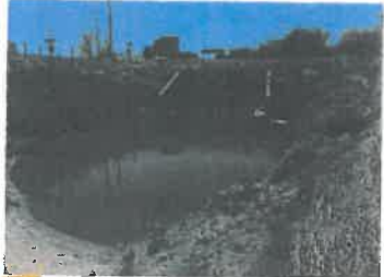
25) The drainage swale from the RC box culvert and 48" RCP drainage structures experienced areas of scour and deposition from the 2019 flood event that impacted its design elevation of 1056.0 feet NGVD29. Excavate floodway to elevation 1055.5, place 6 inches of topsoil to elevation 1056, and seed.
