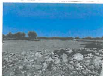
26) The Salt Creek floodway experienced deposition from the 2019 flood event that impacted its design elevation of 1056.5 feet NGVD29. Excavate floodway to elevation 1056, place 6 inches of topsoil to elevation 1056.5, and seed.
