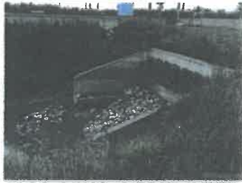
22) Approximately 8 feet of scour downstream of the reinforced concrete box culverts into the riverside levee section and BNSF berm for a length of 75 feet, leading to failure of the erosion control matting and large erosion gullies in the embankment slope. Additionally, there is 3 feet of scour underneath the wingwalls of the drainage structure. See the structural drawings for final repair.
