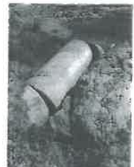
20) The 48" diameter RCP outlet, wingwalls, and footing at station LV 8+60 have fallen into a scour hole in the Salt Creek Floodway. See the structural drawings for final repair.
