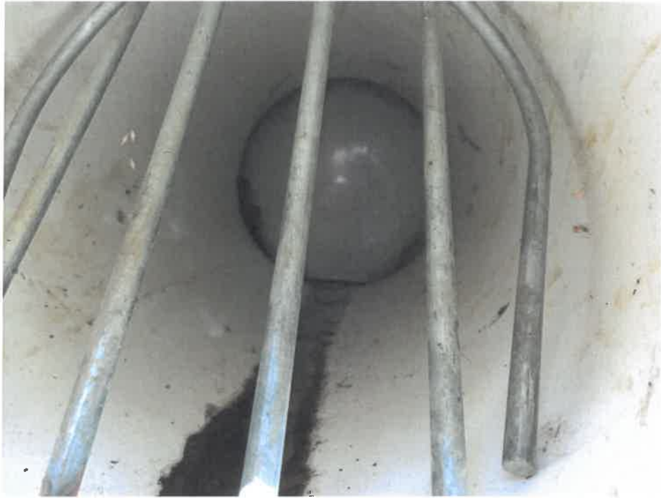
Fig. 4: West outlet pipe with gate closed. (9/6/2019)
