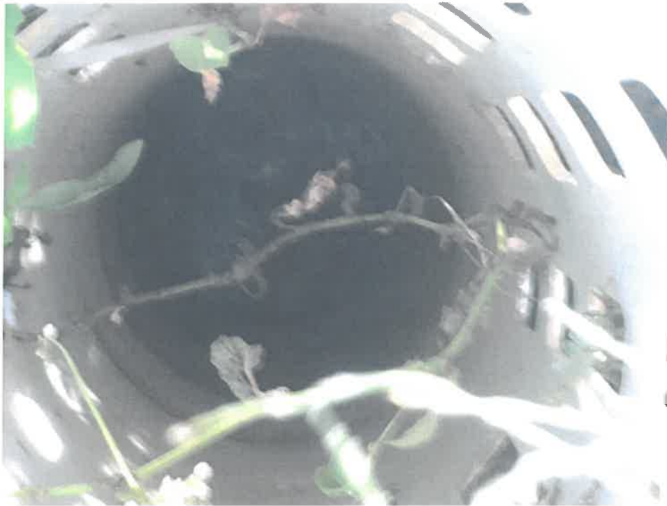
Fig. 10: Looking into west tile inlet on Benes Service Co. property (9/6/2019)
