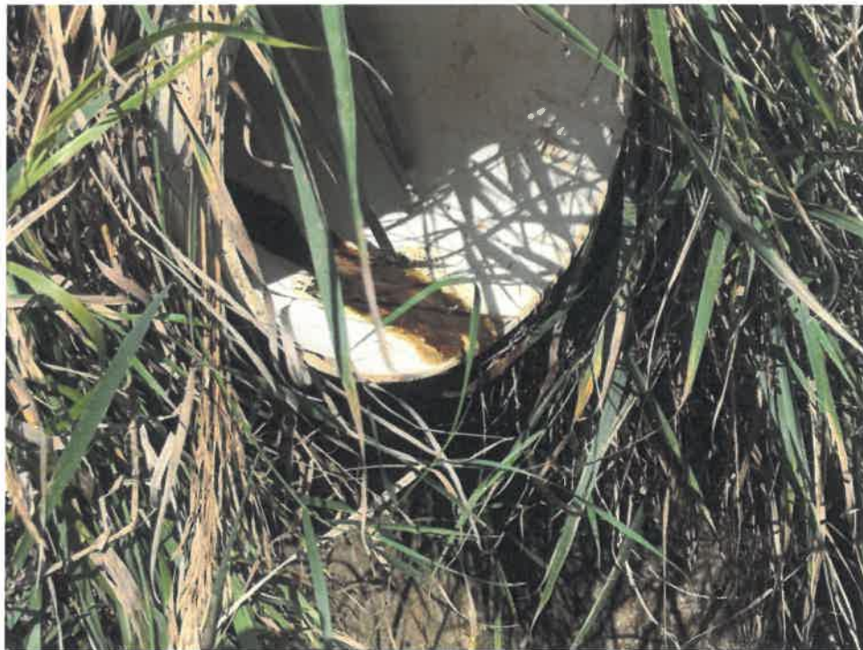
Fig. 3: Close look at far left tile outlet dripping. (9/6/2019)
