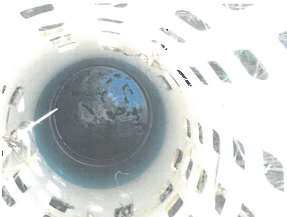
Fig. 9: Looking into middle tile inlet on Benes Service Co. property (9/6/2019)
