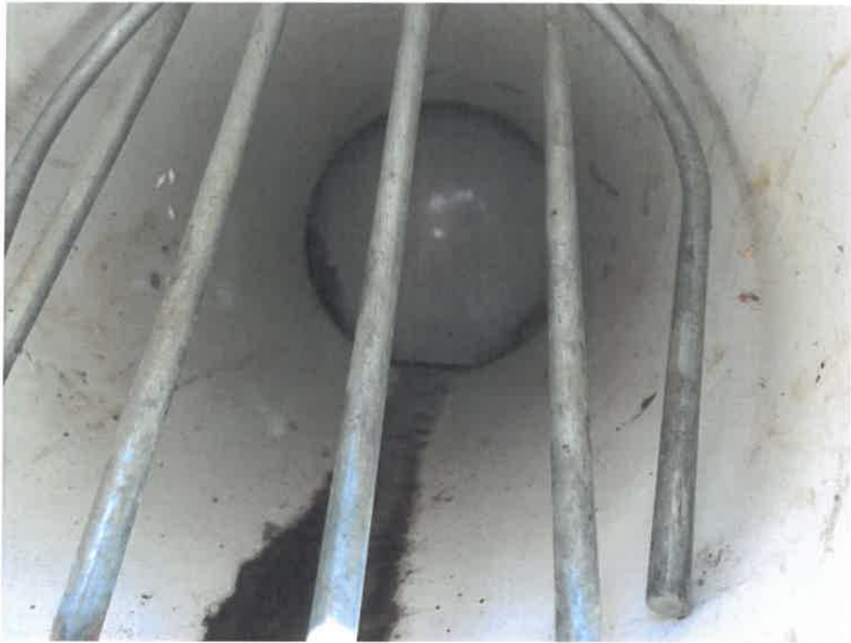
Fig. 4: West outlet pipe with gate closed. (9/6/2019)
