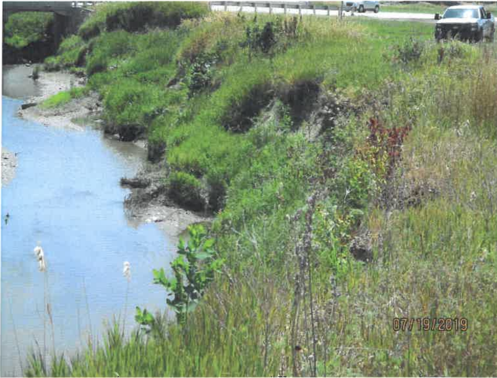
Figure 1: Looking south toward NE 50 bridge.
