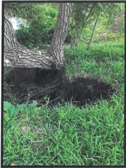
Picture 5 Erosion and failure of
