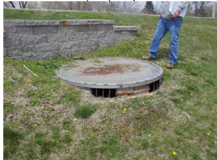
Principal Spillway Inlet
