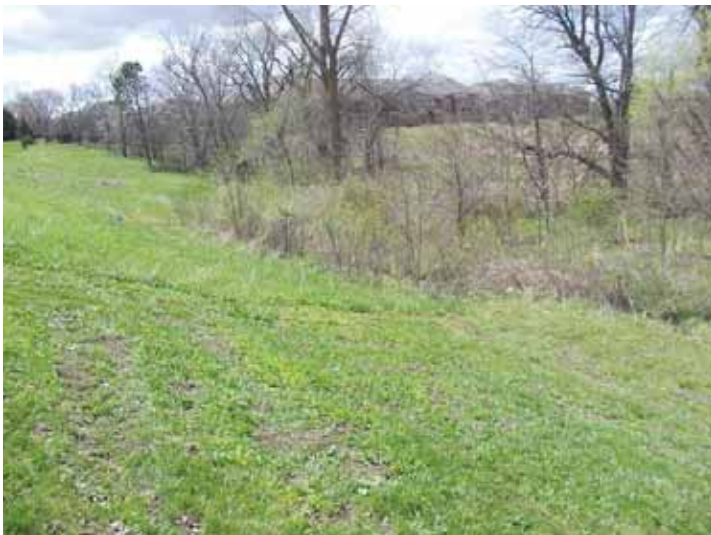
Small trees/brush on downstream toe of dam
