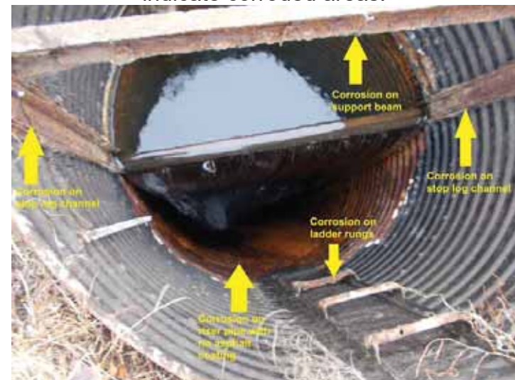
Looking down into principal spillway inlet. The yellow arrows indicate corroded areas.
