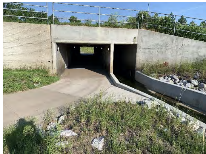
Figure 1: Culvert at 84th & Old Cheney Road
