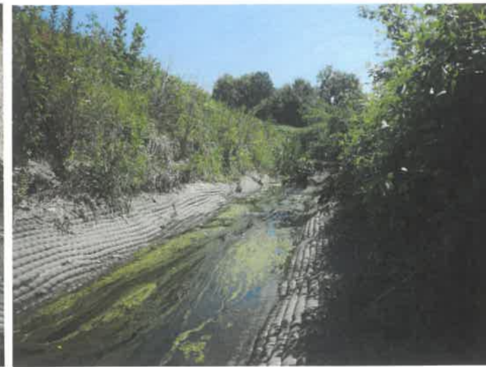
ARTICULATED CONCRETE BLOCK CHANNEL
