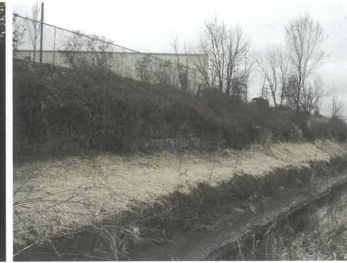
PIPE OUTLET AND GABION WALL
