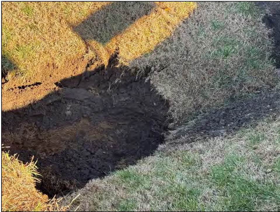
Photo 2: Closeup of sinkhole in road embankment above south culvert.
