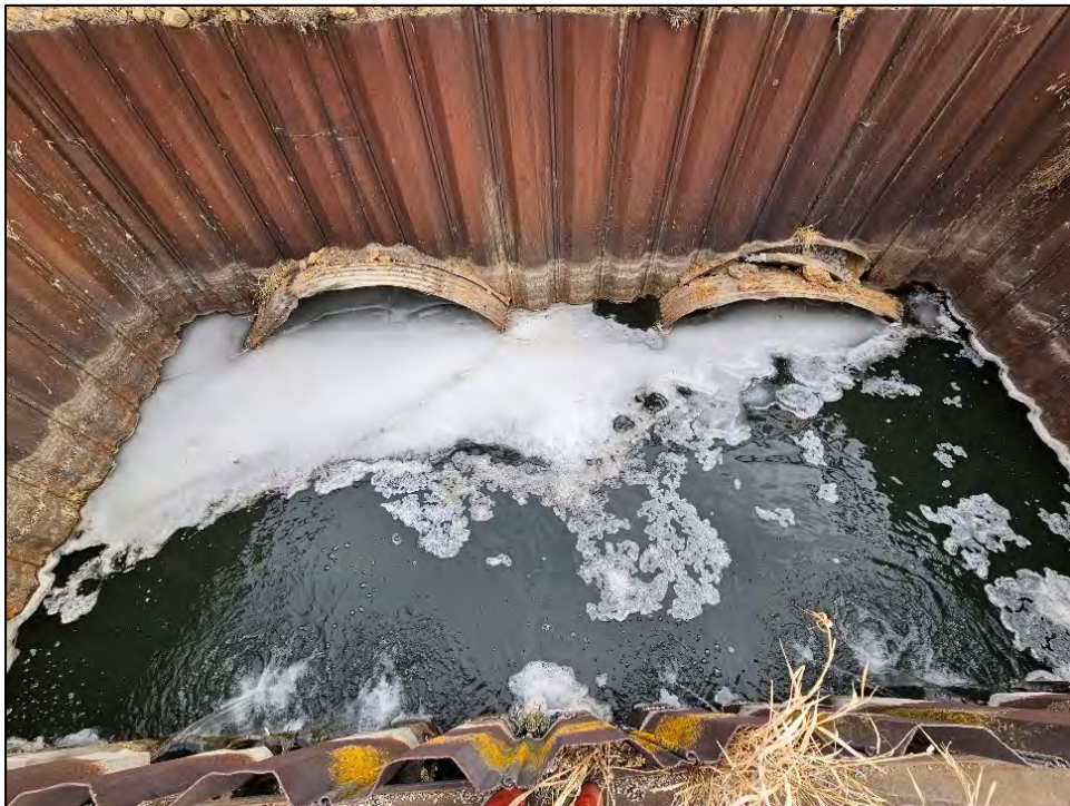
Photo 6: Closeup of upstream end of culverts after temporary emergency repair, with the right (south) culvert showing some deformation at the sheetpile headwall.
