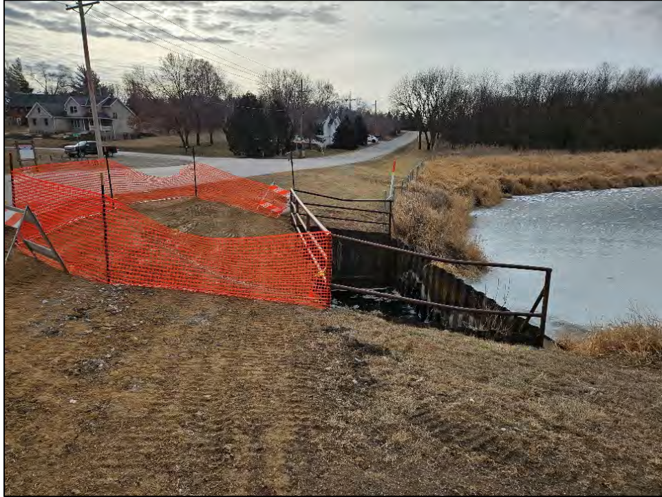
Photo 7: Beaver Lake Boulevard embankment above culvert backfilled in temporary emergency repair
