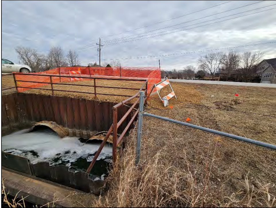
Photo 5: Upstream end of south culvert after sinkhole was filled during temporary emergency repair. The crushed section of pipe remains in place.
