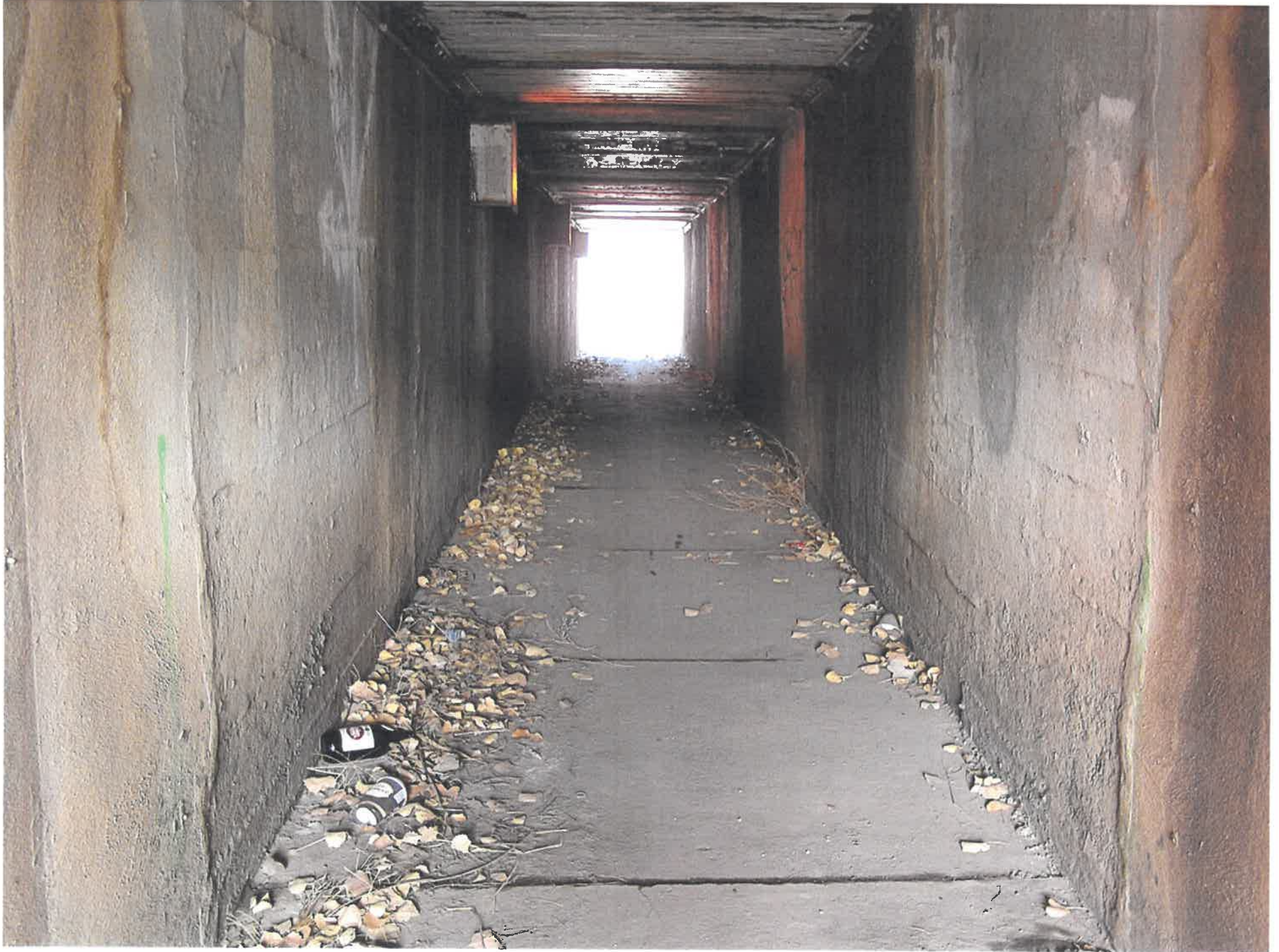
1st & J Street Current Under crossing Box Culvert
