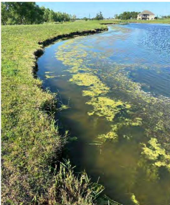
PHOTO 7 (NORTHEAST POND): WEST SHORELINE, LOOKING NORTH
