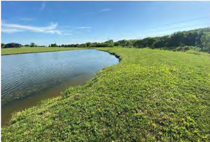
PHOTO 20 (SOUTHWEST POND): NORTH & WEST SHORELINE, LOOKING SOUTHWEST
