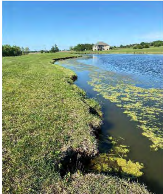
PHOTO 6 (NORTHEAST POND): WEST SHORELINE, LOOKING NORTH
