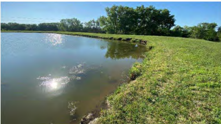
PHOTO 16 (SOUTHWEST POND): EAST & NORTH SHORELINE, LOOKING NORTH
