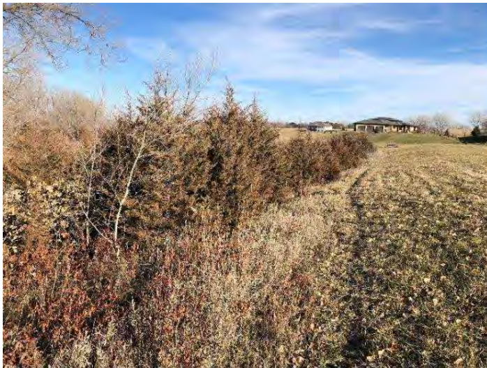
Remove trees on the downstream side of the dams
