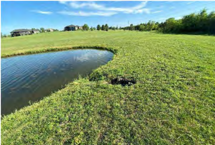
PHOTO 24 (SOUTHWEST POND): WEST SHORELINE, SOUTHWEST LIMITS OF DAM LOOKING SOUTHWEST
