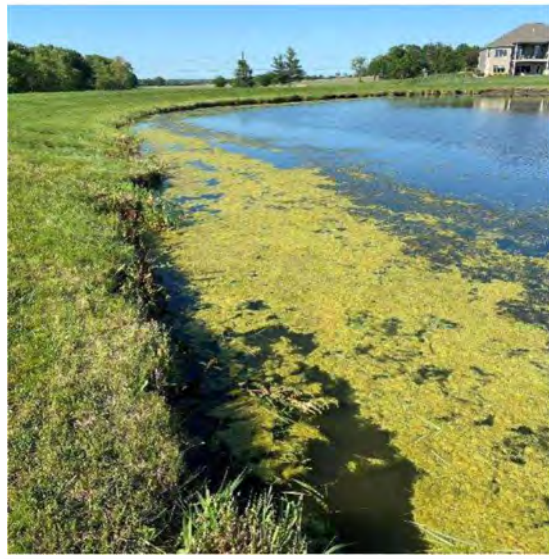
PHOTO 10 (NORTHEAST POND): NORTHWEST CORNER, NORTHERN LIMITS OF DAM, LOOKING NORTH
