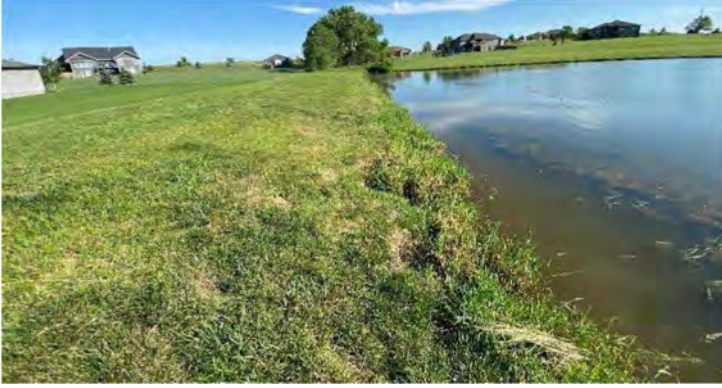
PHOTO 13 (SOUTHWEST POND): EAST SHORELINE, SOUTHEAST LIMITS OF DAM, LOOKING SOUTH
