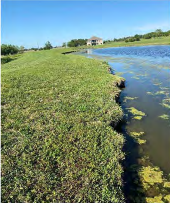
PHOTO 5 (NORTHEAST POND): WEST SHORELINE, LOOKING NORTH
