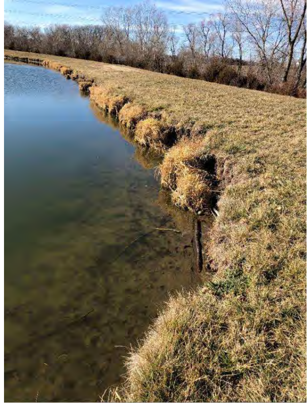
Repair and reinforce damaged areas on both dams
