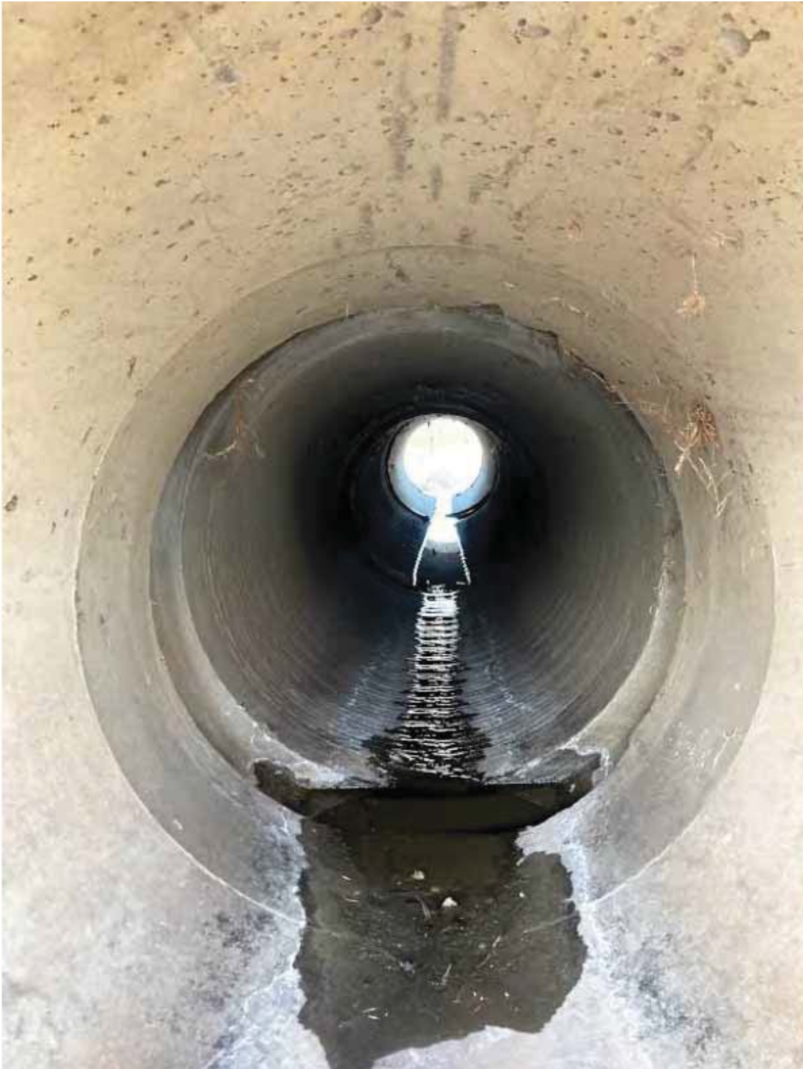
RIGHT CULVERT LOOKING NORTH
