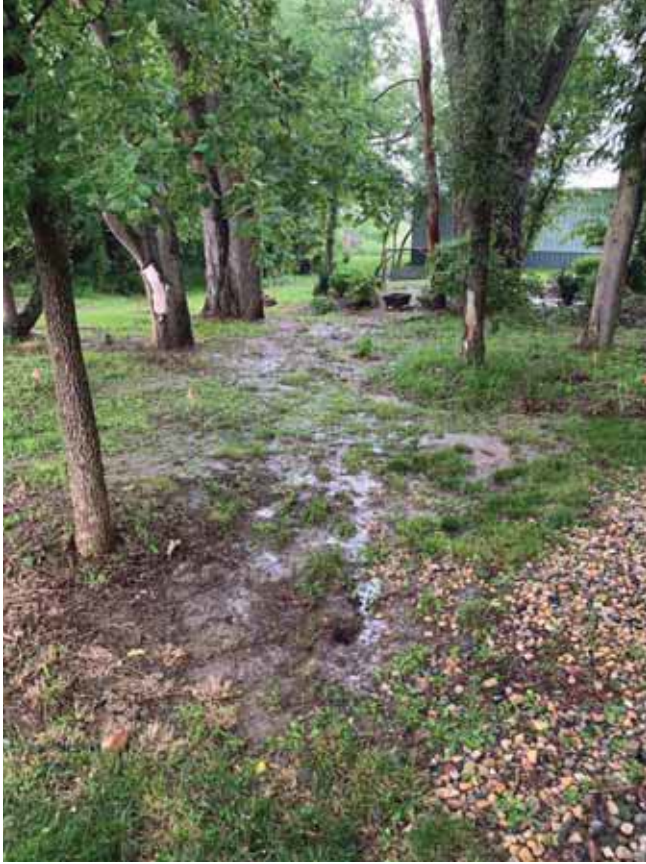
Creek 1: View of general drainage/water issues heading toward main Creek 1 flow.
