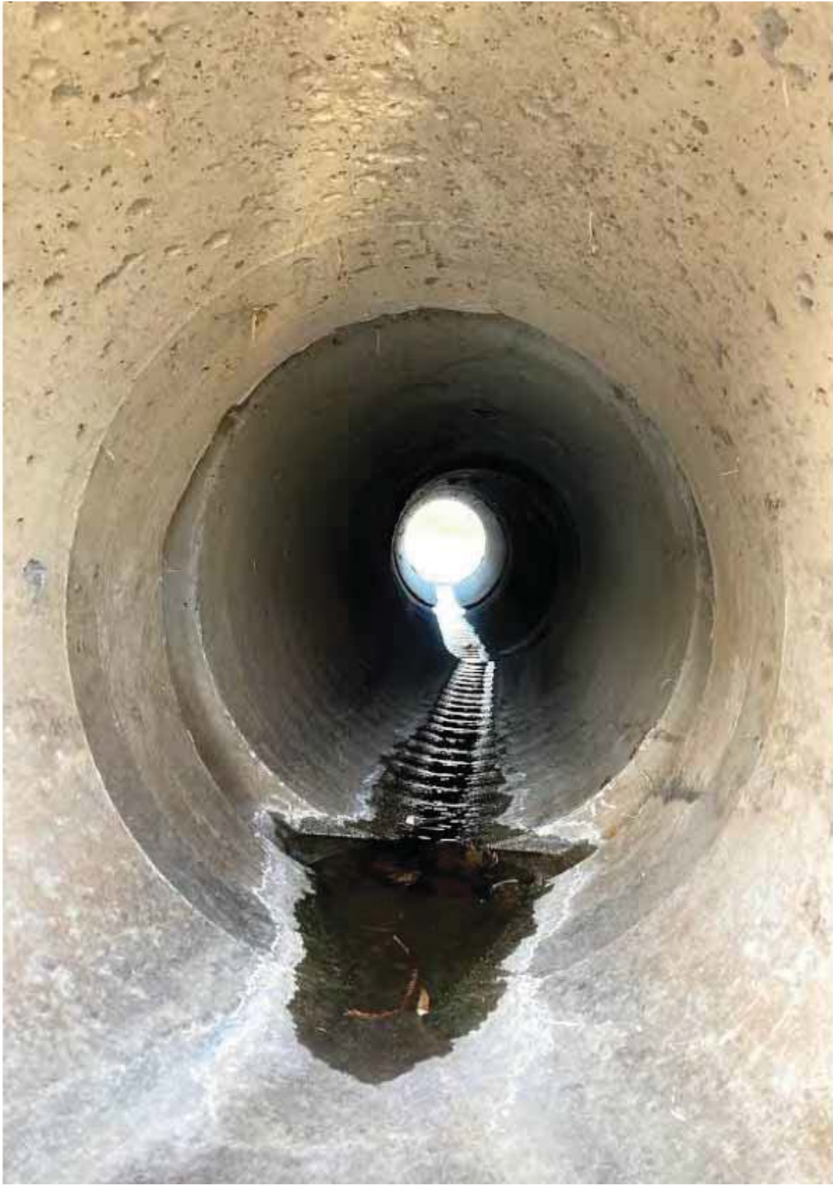
LEFT CULVERT LOOKING NORTH
