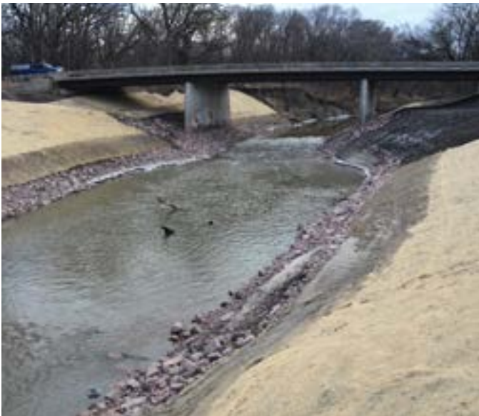
This recent stream stabilization project on Salt Creek at Pioneers Boulevard, in Wilderness Park, is part of the South Salt Creek Watershed Master Plan. To learn more about this interesting project and about the benefits of watershed master planning in Lincoln, see the article on page 6.
