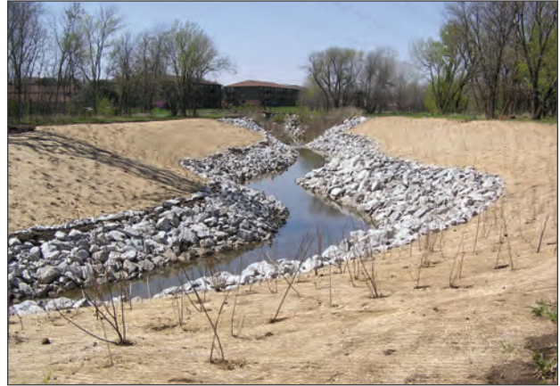
Urban stream improvement
