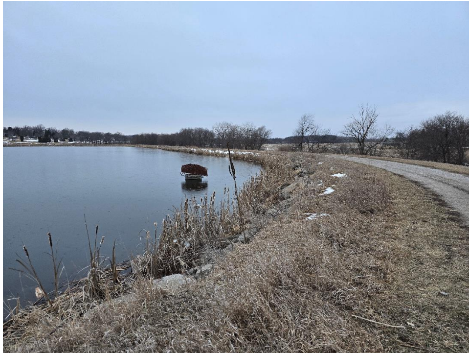
Figure 1: Spillway Riser and Top of Dam (JEO Site Visit, February 25, 2026)
