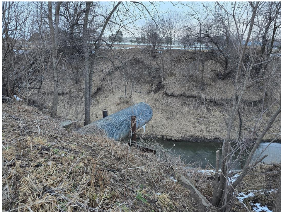
Figure 2: Spillway Outfall (JEO Site Visit, February 25, 2026)
