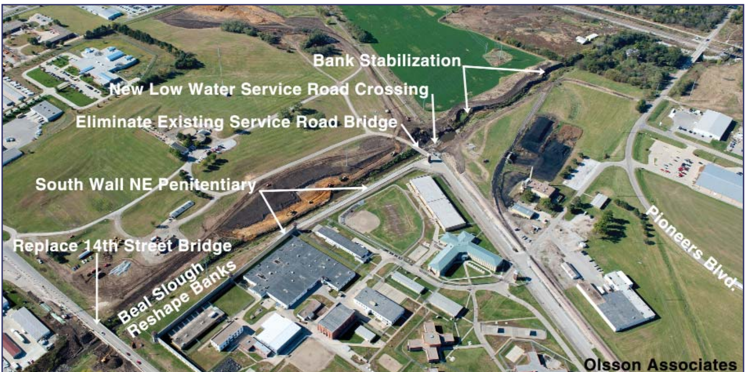
Beal Slough Project near Nebraska Penitentiary
