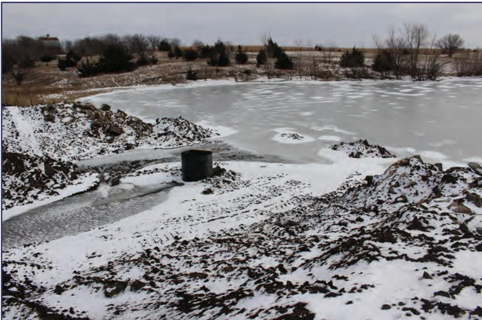
*The riser that controls the level of Upper Salt Dam 18-9, near Princeton, has been replaced after it was damaged in storms last spring, but work still remains.*
